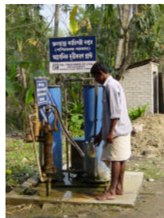
Picture 2: Arsenic Removal Filter Mogra Bazar, Kamdebkathi
