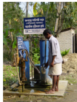
Picture 2: Arsenic Removal Filter Mogra Bazar, Kamdebkathi
