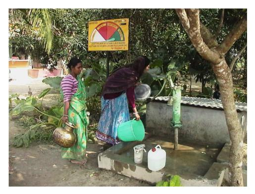
Fig. 1. Newly installed shallow dugwell with hand pump extraction of water to replace tubewell with water arsenic concentration of  $220 \mu g/l$ . Arsenic concentration in this dugwell was  $6 \mu g/l$ , but concentrations in such dugwells may be in range from 2 to  $50 \mu g/l$ .
